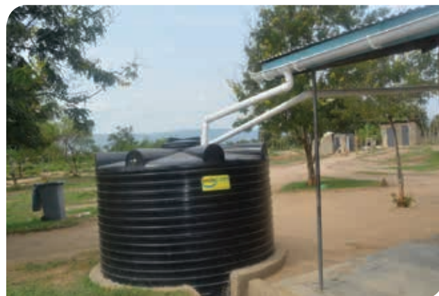
Above; the 10,000 litre tank that was installed at the Maternity Ward at Morulem Health Centre in Abim. Below Paediatric Ward at Kyango Health Centre Kalisizo;
